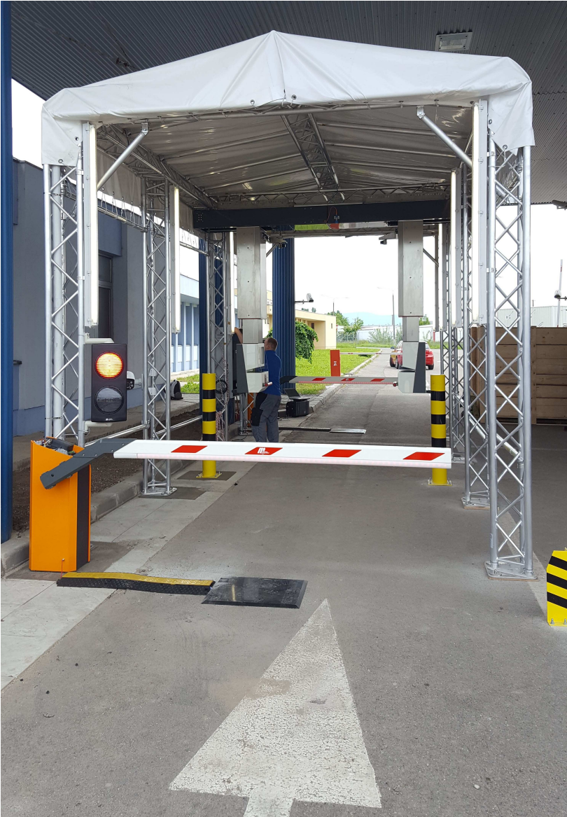
Test installation at Moravita - © Magnetic Autocontrol Group
